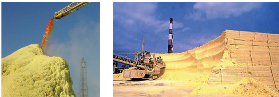
Figure 1 – Example of conventional open air sulfur storage (Lacq field – South West France)
